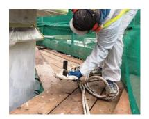
Homeshield in consultation with Wetherby Stone Products specified **Wethertex GRC backing coat render, a fibre re-enforced, high-polymer trowel applied render** which is designed to adhere well to difficult substrates and act as a water-proofing backing coat for subsequently applied decorative finishes. **Upvc angle corner/angle beads** were used to prevent the likelihood of any future corrosion.
